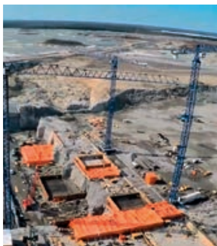
22 Telebelt at Keeyask Project in Canada
