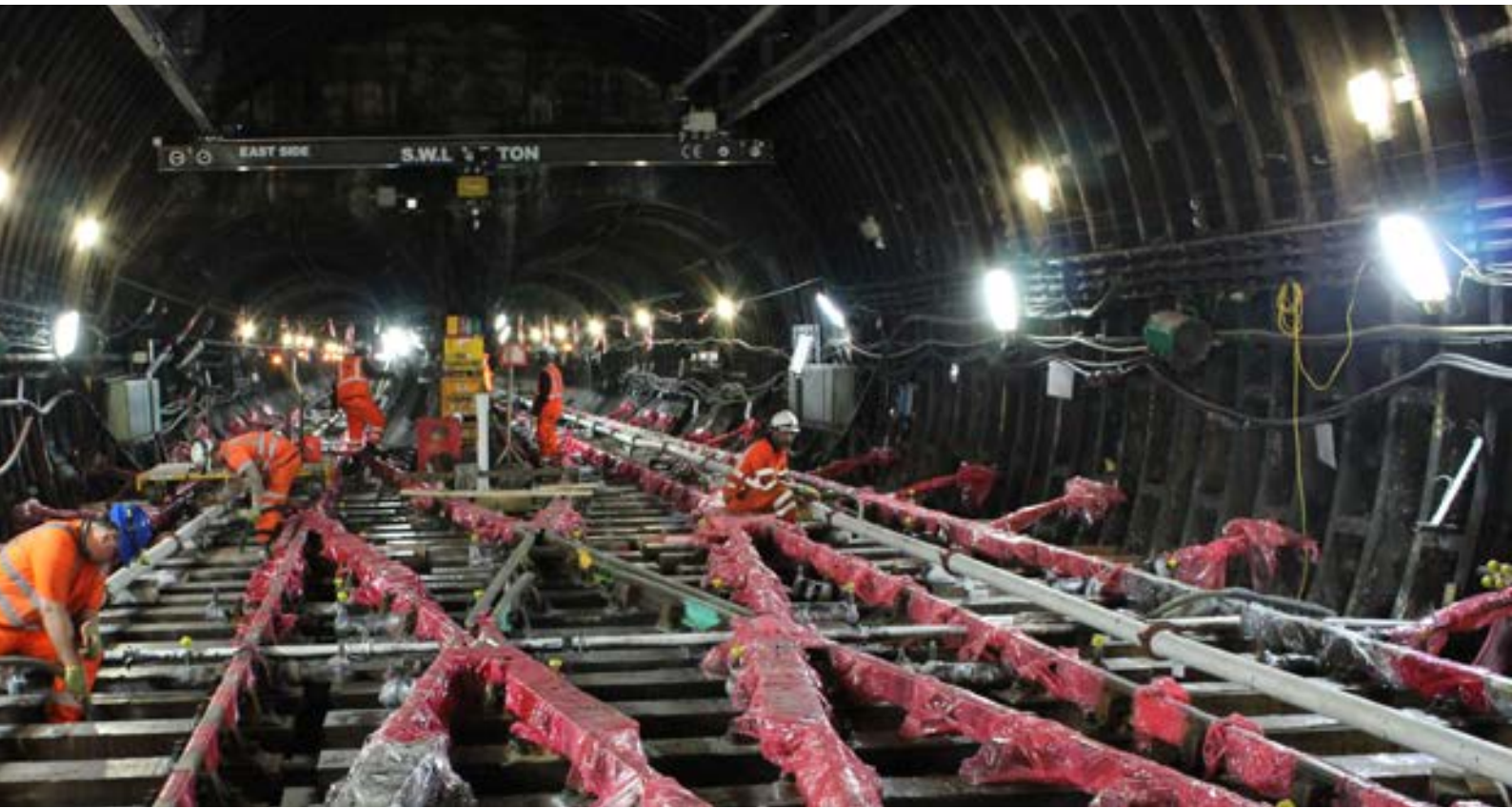
Installing the pipelines in the cavern
