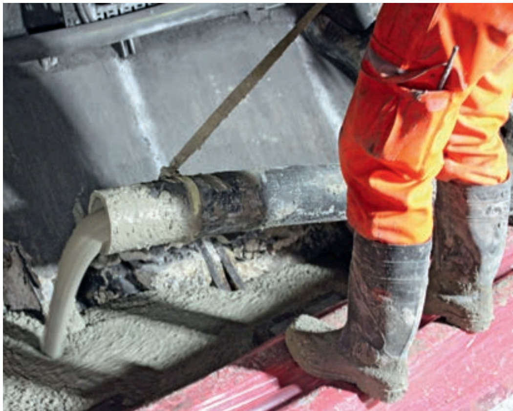
Concrete flowing into the trackbed
