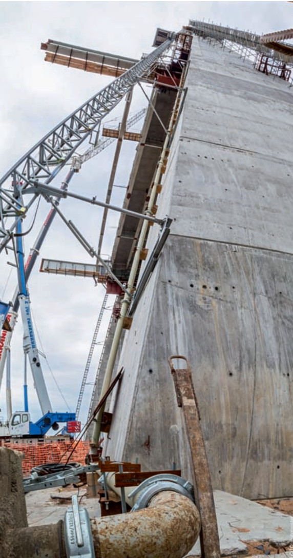
▲ Concrete was pumped up to a height of approx. 96 m using SK delivery lines
