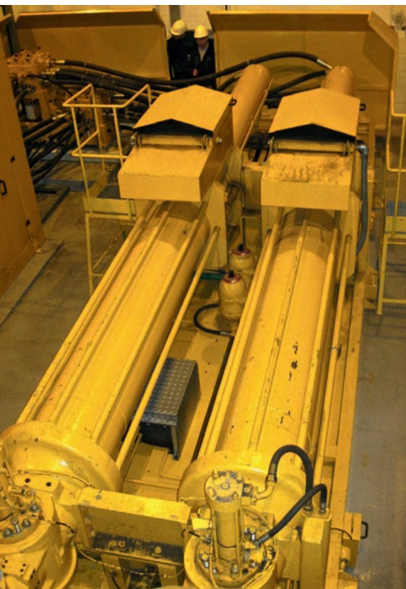
▲ Two of the six HSP 25150 HP pumps in Belchatow power station
