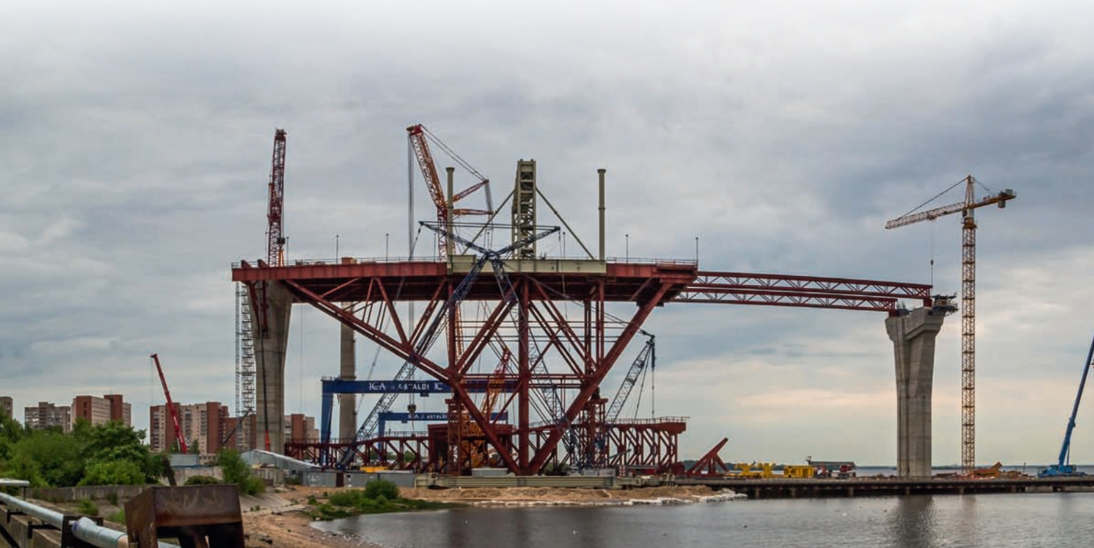
▲ Concrete was pumped up to a height of approx. 96 m using SK delivery lines
